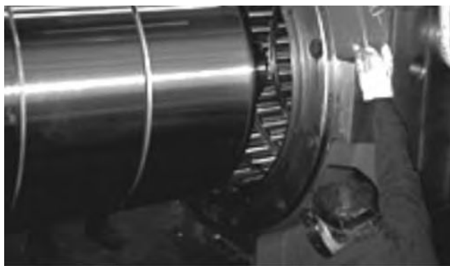
Fig. 255. Installing chock assembly onto roll neck and inner ring.
