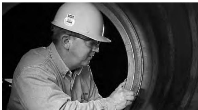
Fig. 238. Polishing out chock bore corrosion.
