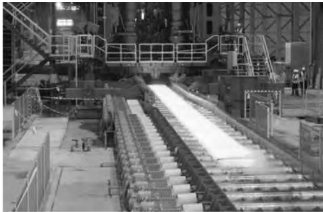
Fig. 113. Hot-strip mill transfer roller table.
